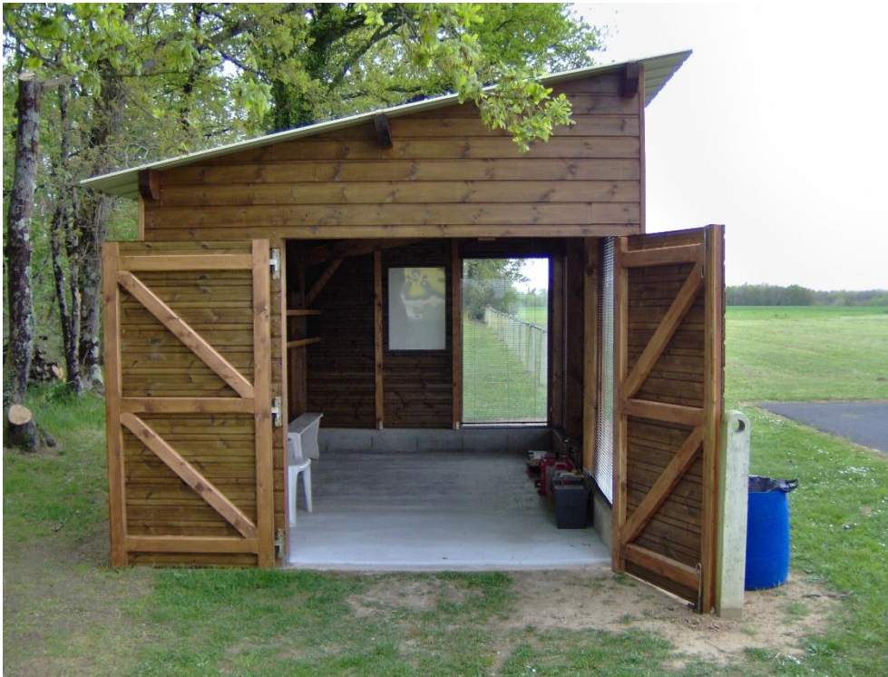
Room for entering notes equipped with an electrical panel for charging batteries
